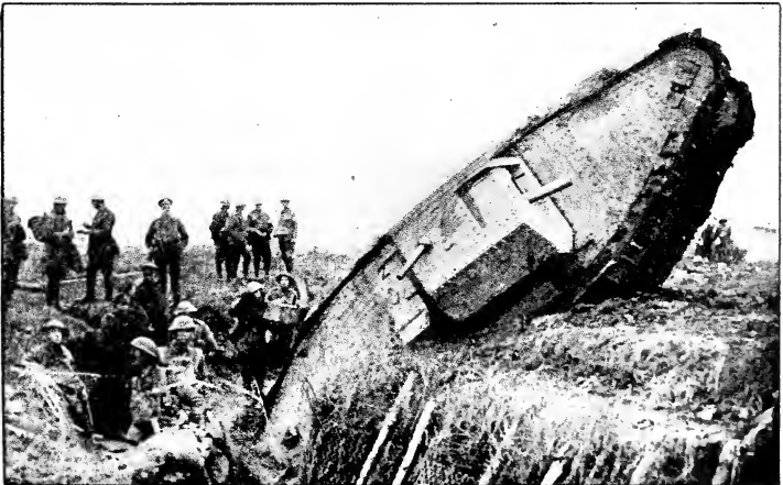
FAILURE OF A TANK TO CROSS A TRENCH
